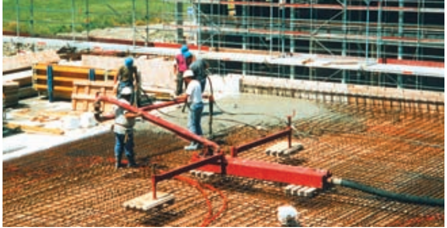
The rotary distributor RV 7: Weight without ballast 610 kg · ballast 280 kg
